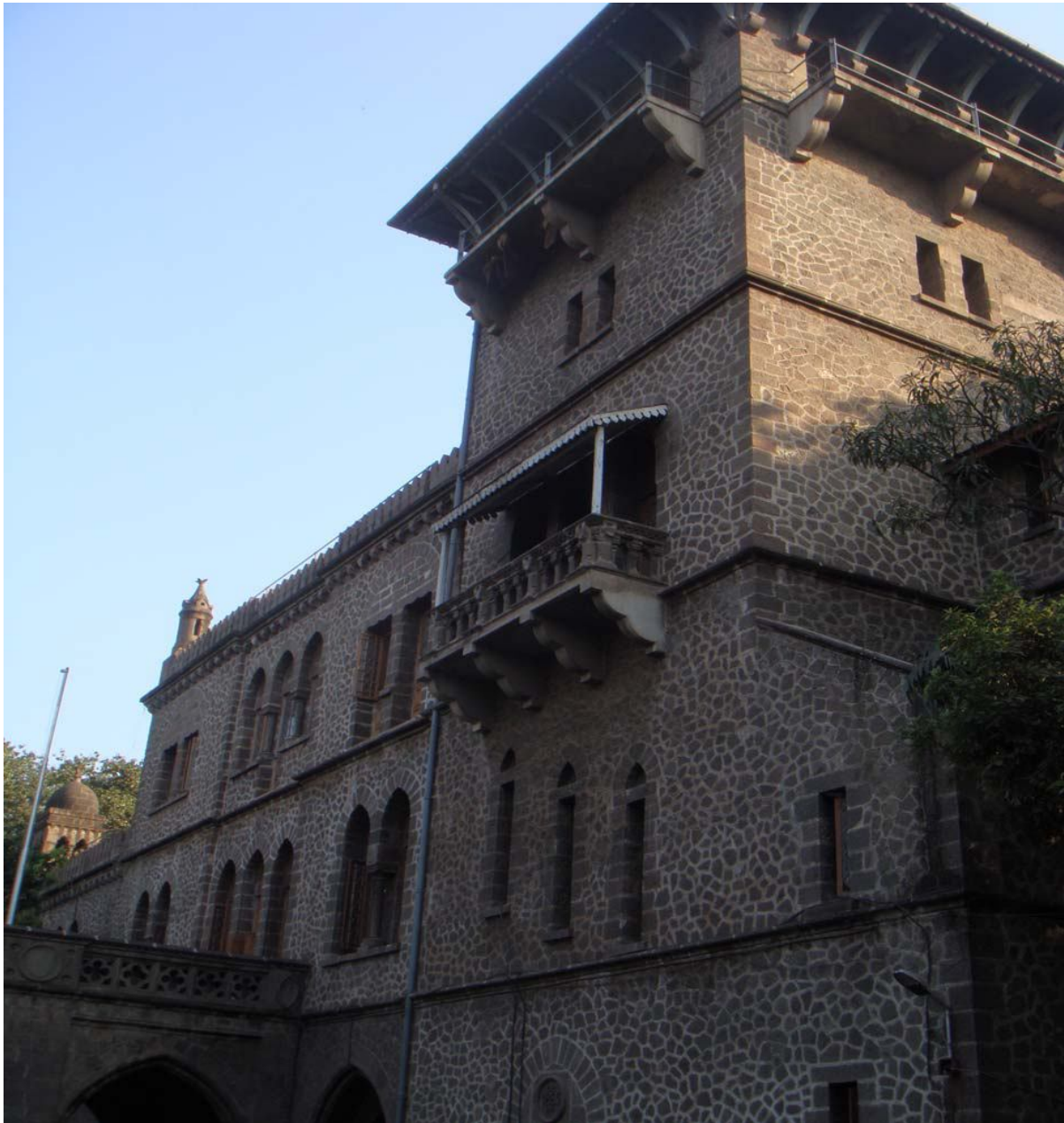
College of Engineering, Pune – 411 005
